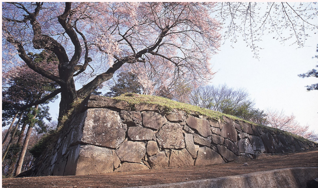
御殿桜と西櫓台石垣 /Goten-sakura and the stone walls of Numata Castle
